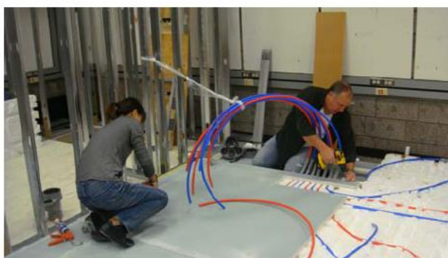
MATRIX TILE SYSTEM installation with 0-slope gray water drains
